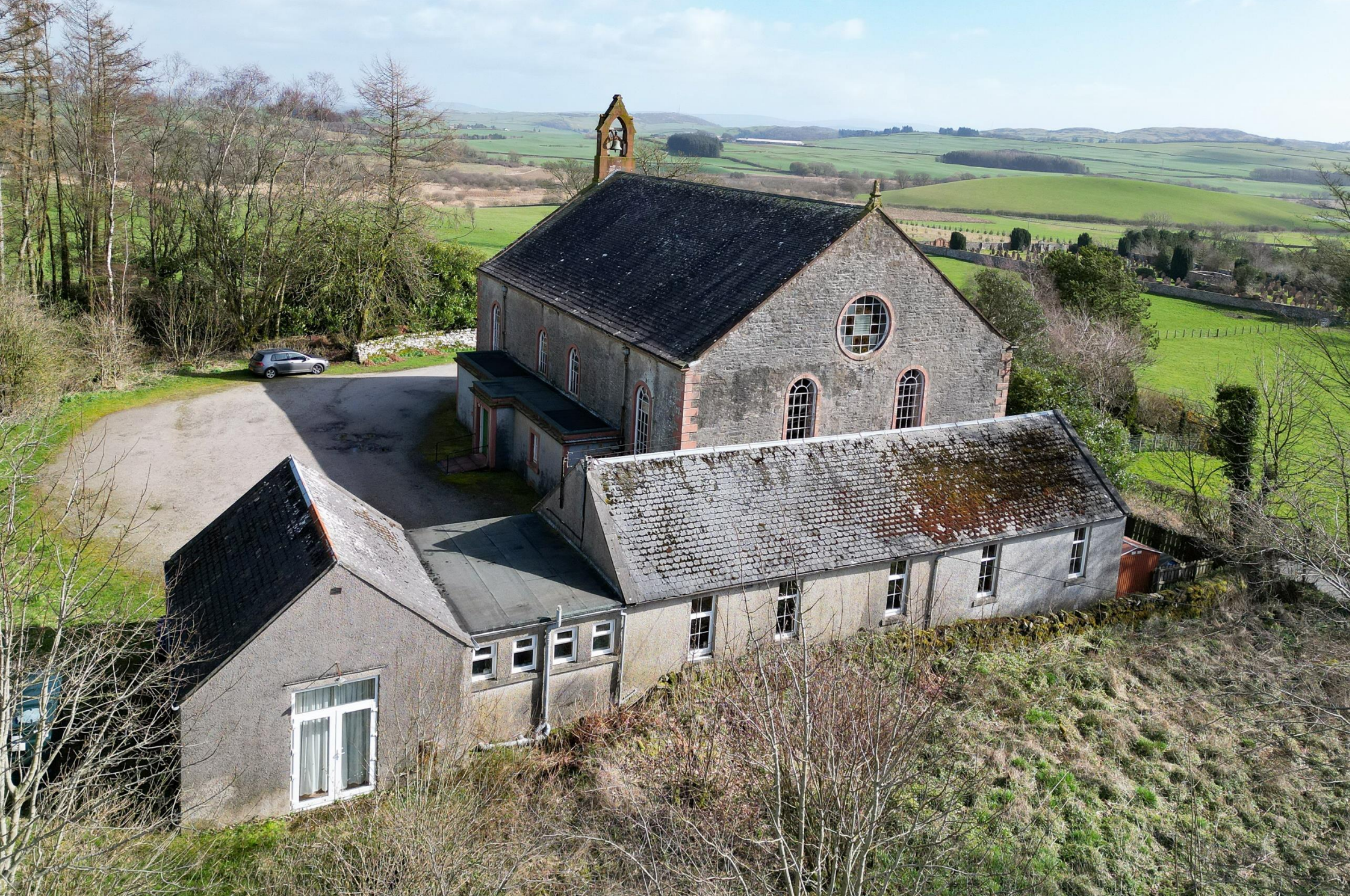
Kelton Church and Hall, Kelton, Castle Douglas, DG7 1RX
