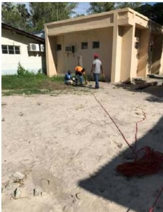
Pegging out the foundation of the oxygen housing
