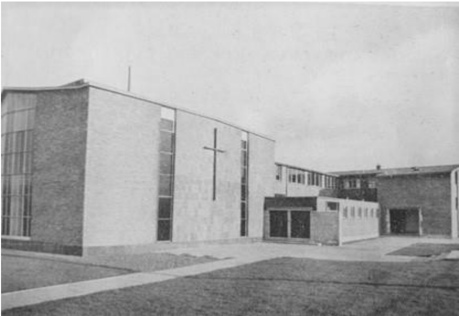
Completed church with grounds laid out circa 1958
